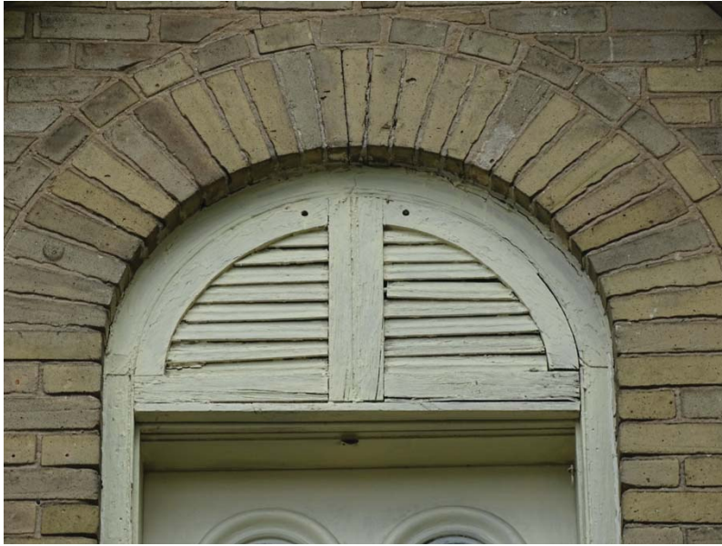
Figure 32: Exterior Transom/Shutter above Second Floor Door
