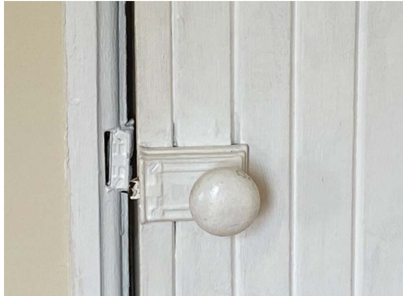
Figure 43: Rim/Box Lock and Ceramic Knob
