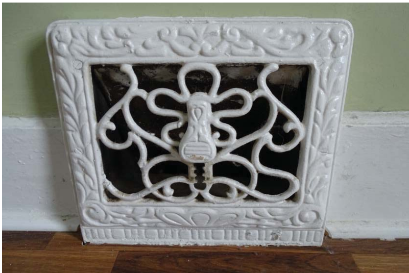
Figure 44: Wall Register
