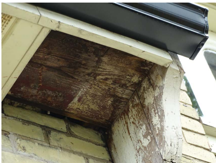
Figure 27: Missing Soffit Section along Front Elevation
