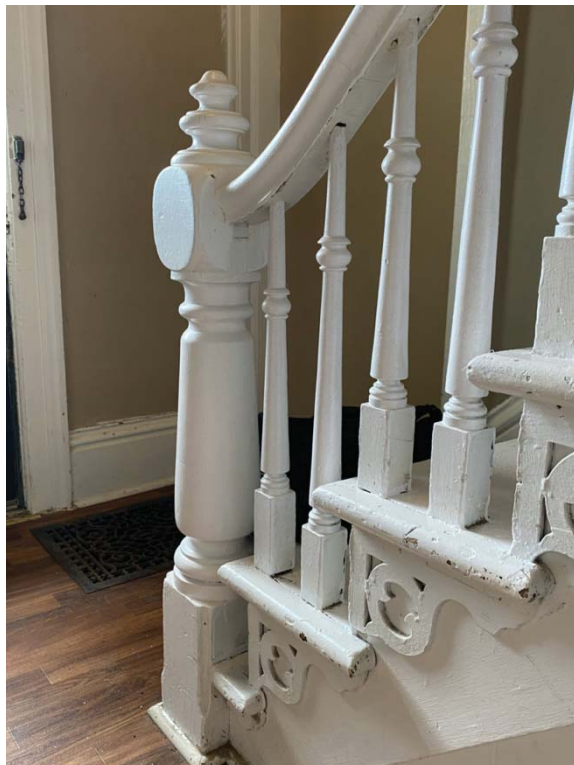
Figure 37: Painted Stair Newel Post and Handrail
