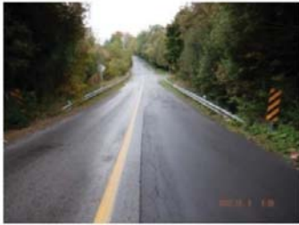
Looking East Over Structure
