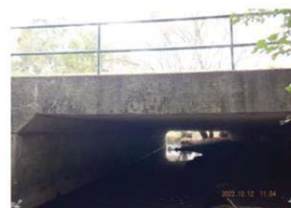
Headwall West Side
