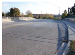
Looking South Over Structure
