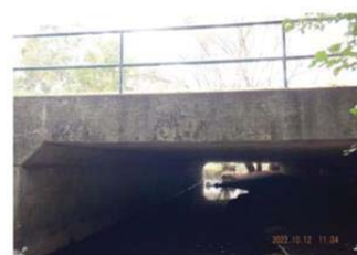
Headwall West Side
