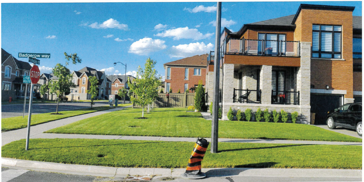
PHOTO 02 - FRONT ELEVATION (SOUTH, FACING BADGEROW WAY)
