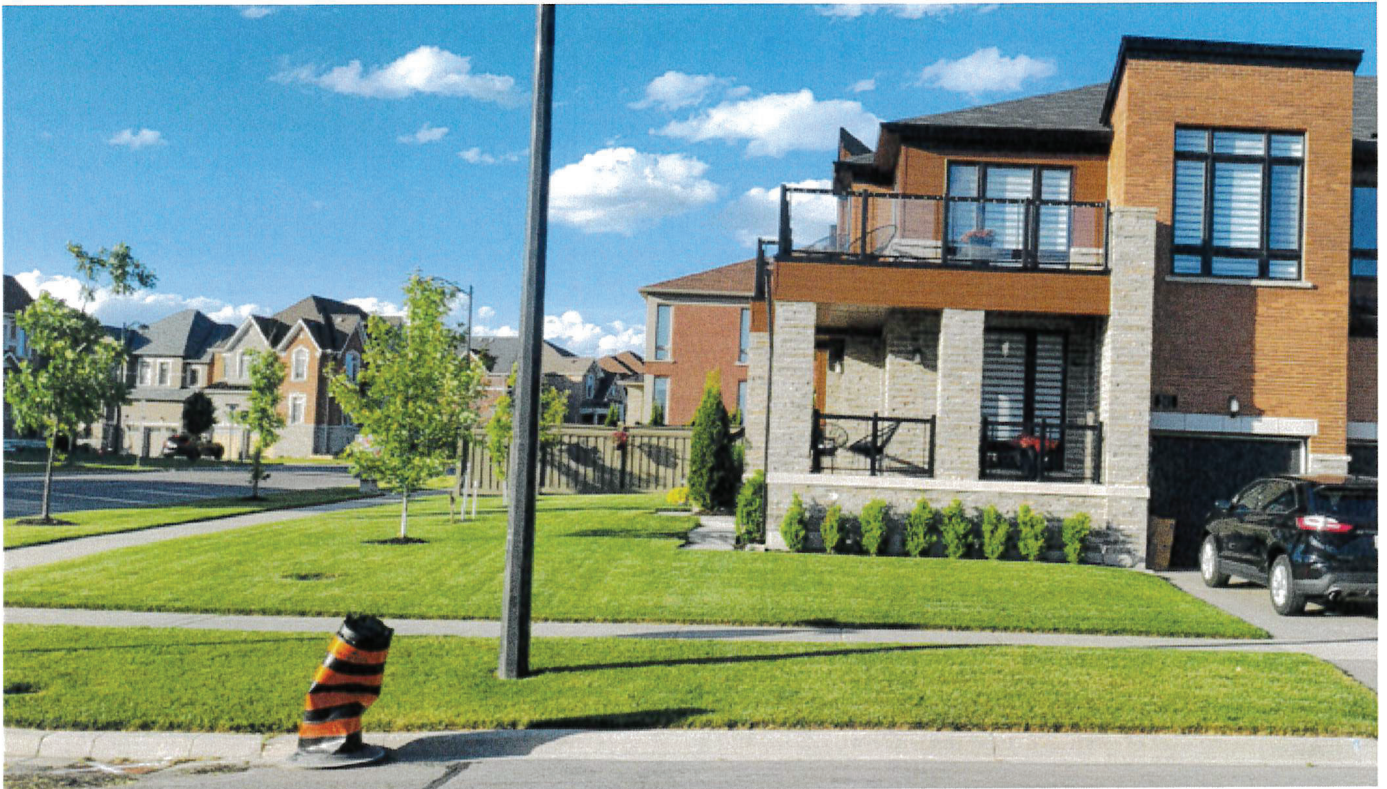
PHOTO 01 - FRONT ELEVATION (SOUTH, FACING BADGEROW WAY)
