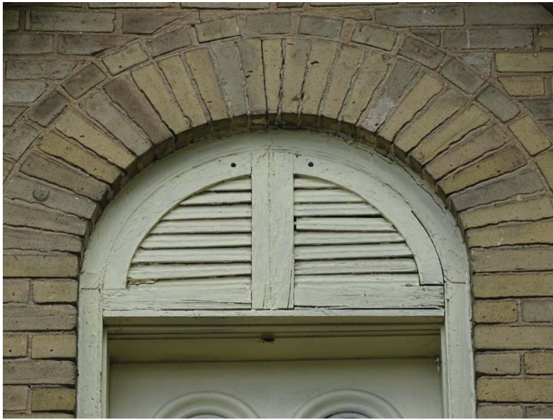
Figure 32: Exterior Transom/Shutter above Second Floor Door
