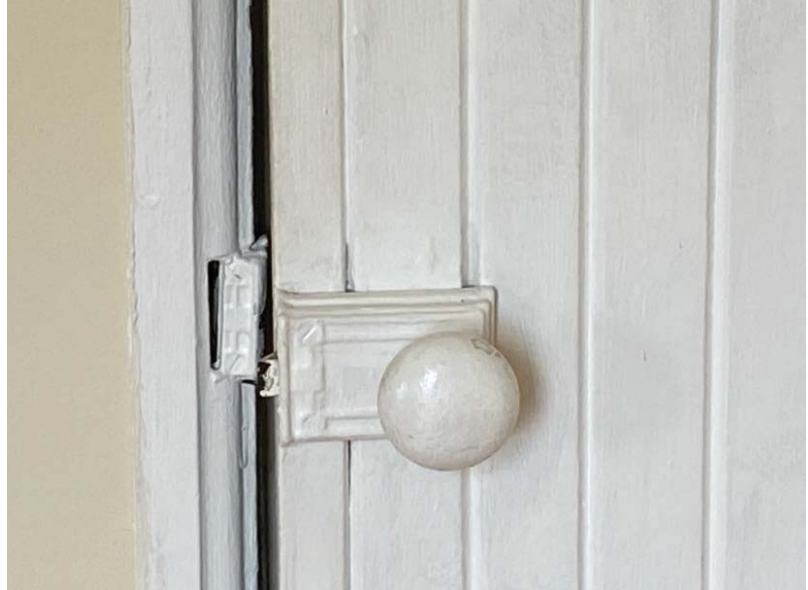
Figure 43: Rim/Box Lock and Ceramic Knob
