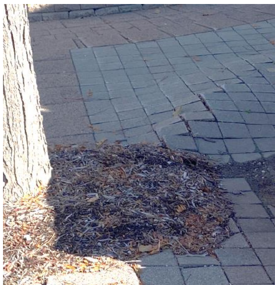
Figure 1 Example of existing pavers in need or replacement
