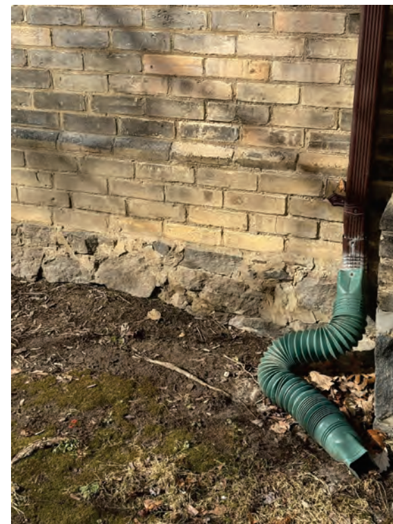
Condition of lower buff brick wall and downspout area
