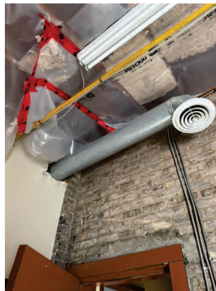
Exposed services, and insulated ceiling assembly against historic brick
