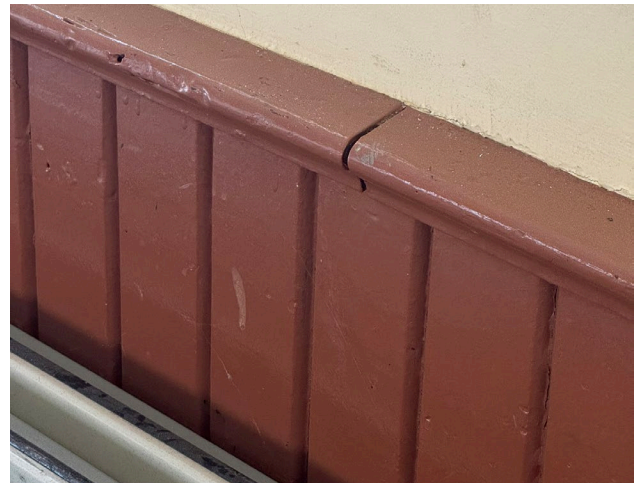
Fig. 5.23. Interior wood wainscoting
