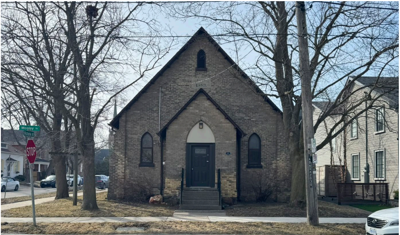
Fig. 1.6. North (principal) elevation facing Mosley Street
