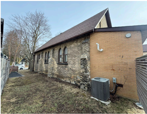
Fig. 5.1. West elevation showing overall wall condition
