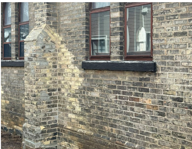
Fig. 5.3. West elevation, typical buttress condition and localized masonry weathering
