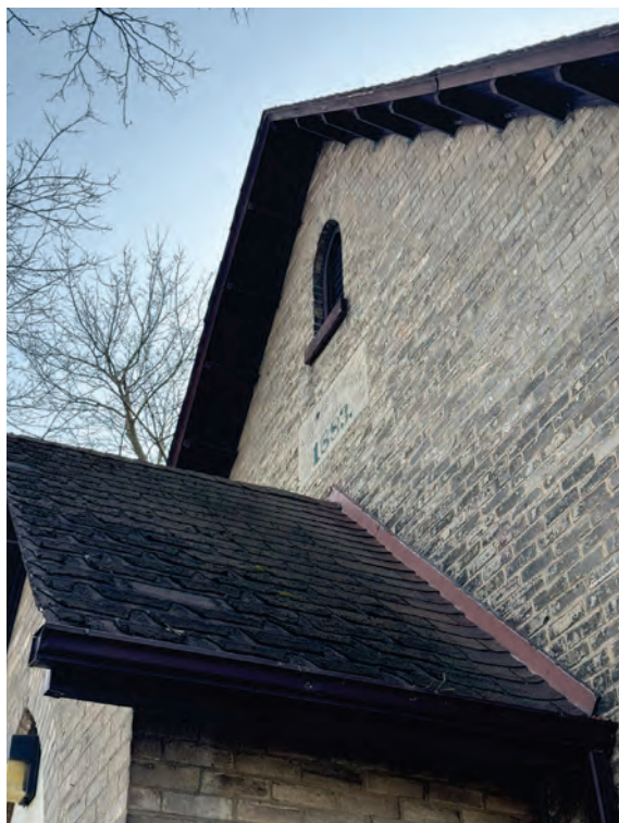
General view of gable end and roofline
