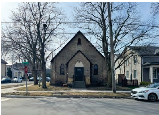
North (principal) elevation facing Mosley Street
