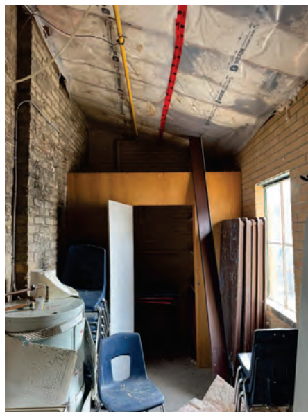
Ancillary space showing alterations, and exposed utilities (current south elevation addition)
