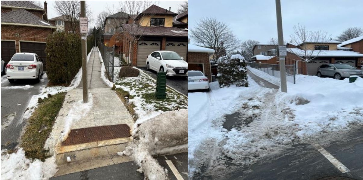
Figure 4 – images of the challenges in plowing this walkway due to a streetlight being installed in the middle of this walkway at both ends:
