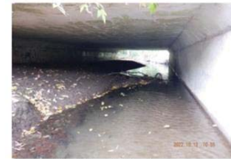
Looking West Through Barrel
