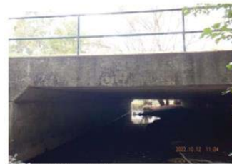
Headwall West Side
