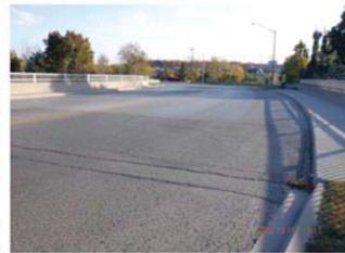
Looking South Over Structure
