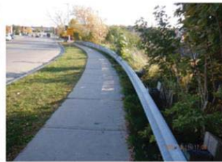
Looking to South SBGR
