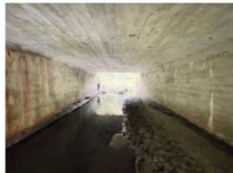
Looking South Through Barrel
