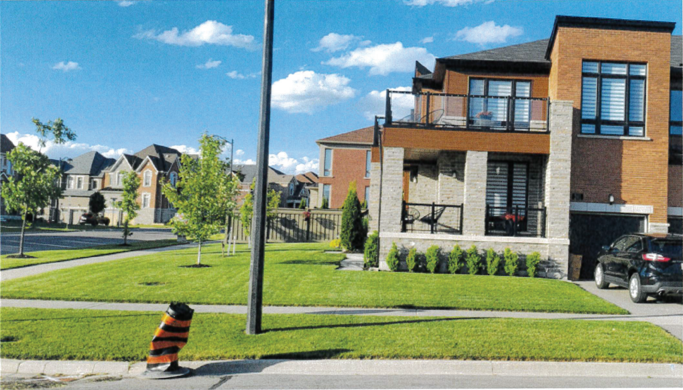
PHOTO 01 - FRONT ELEVATION (SOUTH, FACING BADGEROW WAY)
