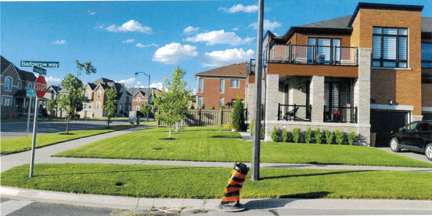
PHOTO 02 - FRONT ELEVATION (SOUTH, FACING BADGEROW WAY)
