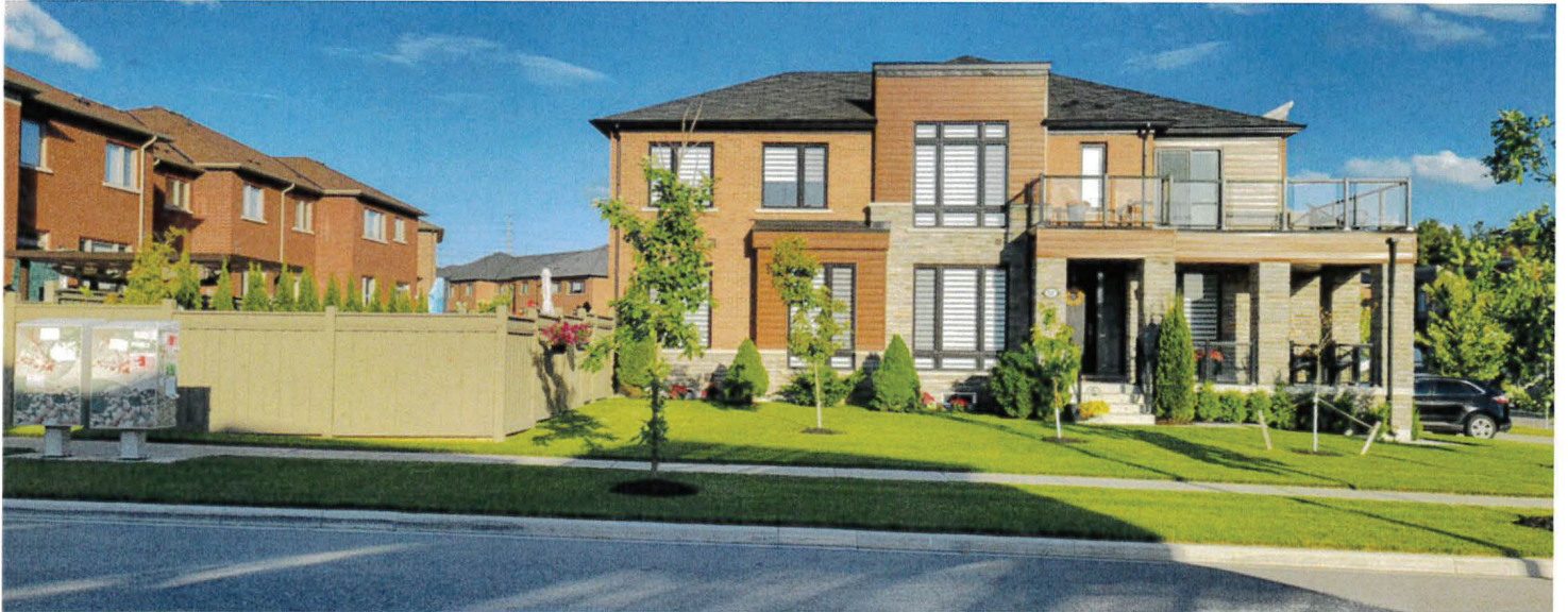
PHOTO 03 - FRONTAGE (WEST ELEVATION, FACING HOLLADAY DRIVE)
