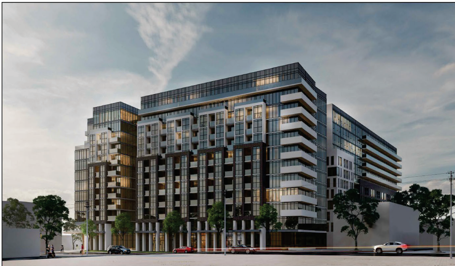
Looking northwest from Wellington Street East
