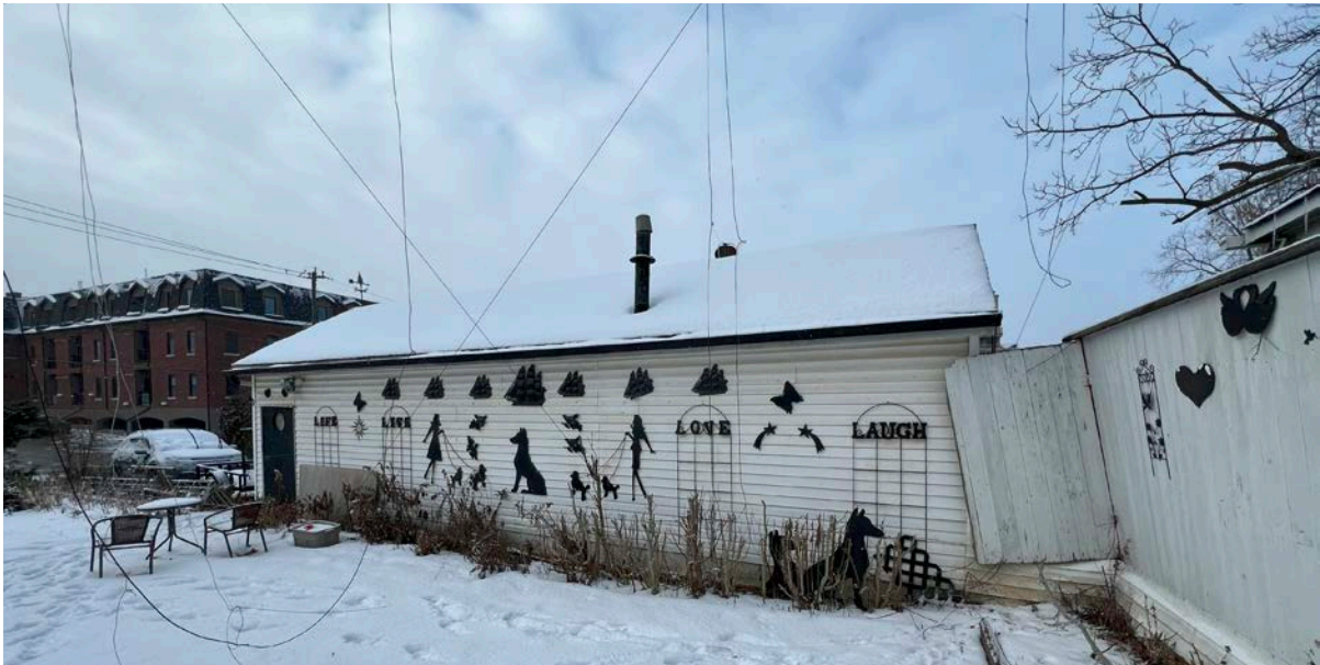
The one-storey garage on the Site, located behind the dwelling (ERA, 2025).
