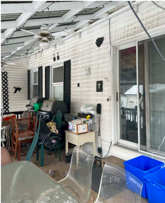
Covered porch at the rear (west) elevation (ERA, 2025).
