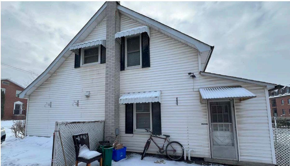
Side (north) elevation of 10-12 Spruce Street. The main entrance to the smaller of the two units in the dwelling is located at this elevation (ERA, 2025).
