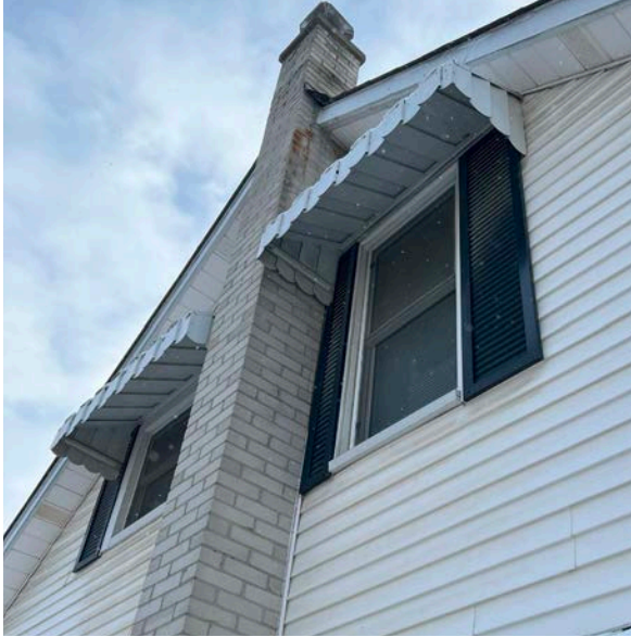
Close-up photo of the side (north) elevation with masonry chimney (ERA, 2025).
