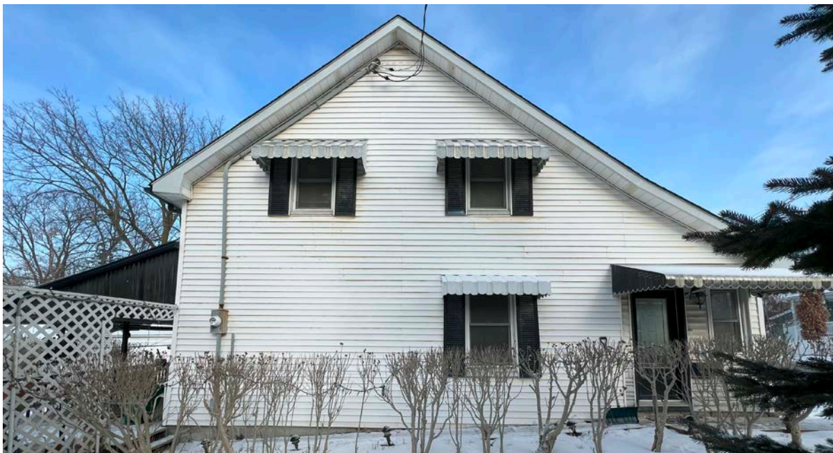
Side (south) elevation of 10-12 Spruce Street. The main entrance to one of the two units in the dwelling is located at this elevation (ERA, 2025).
