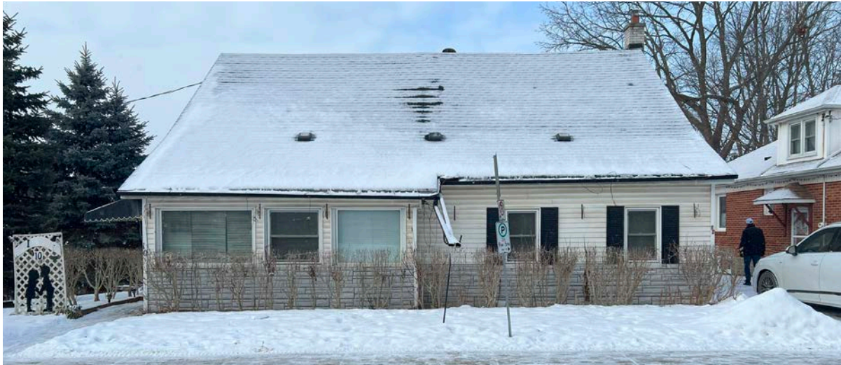
Principal (east) elevation of 10-12 Spruce Street (ERA, 2025).
