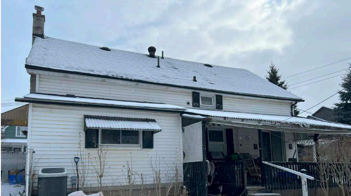
Rear (west) elevation of 10-12 Spruce Street (ERA, 2025).
