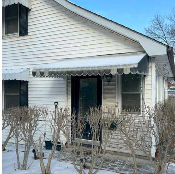
Close-up photo of the side (south) elevation showing the main entrance door to one of the two units in the building (ERA, 2025).
