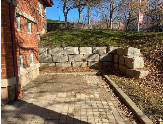
Figure 2 Erosion impacting the armour stone retaining wall on the southeast side of Town Hall
