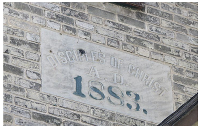
Fig. 2.2. Victoria Hall, Built 1883
