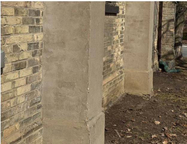
Fig. 5.14. East elevation, buttresses with parged finish
