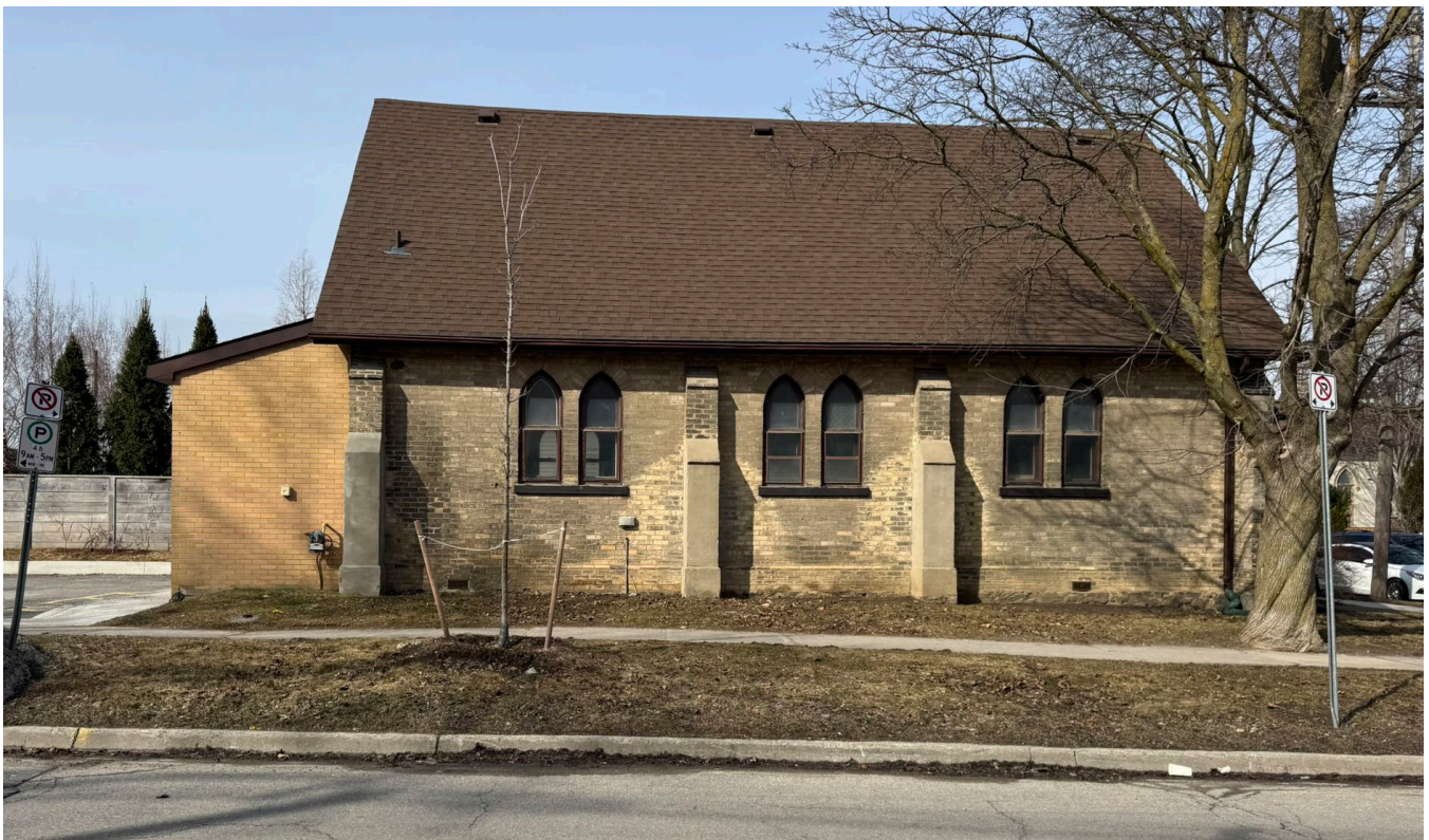
Fig. 1.7. East elevation facing Victoria Street
