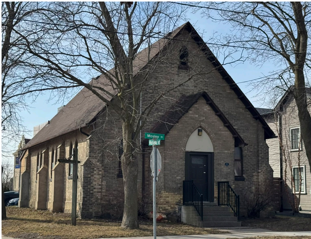
Fig. 2.5. Present-day image of the northeast corner; the exterior remains largely unchanged.
