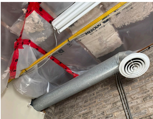
Fig. 5.20. Exposed services, and insulated ceiling assembly against historic brick wall
