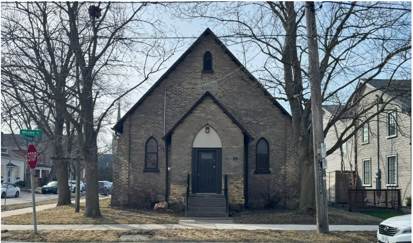
Fig. 1.6. North (principal) elevation facing Mosley Street
