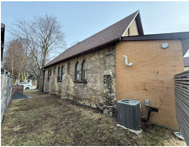
Fig. 5.1. West elevation showing overall wall condition
