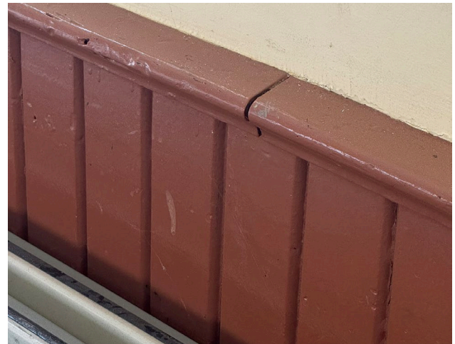
Fig. 5.23. Interior wood wainscoting
