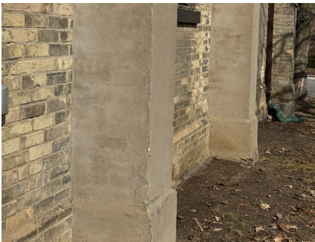
Fig. 5.14. East elevation, buttresses with parged finish
