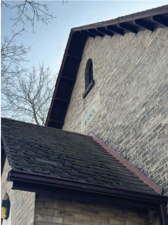
General view of gable end and roofline
