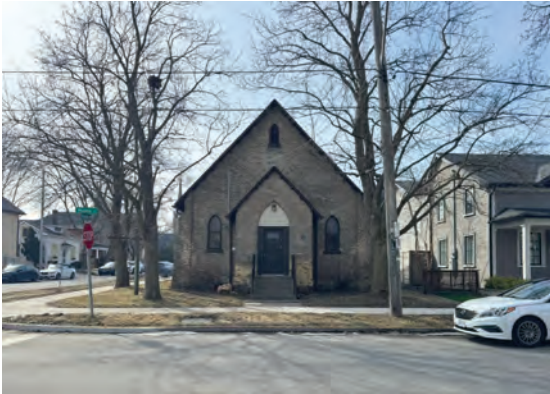
North (principal) elevation facing Mosley Street
