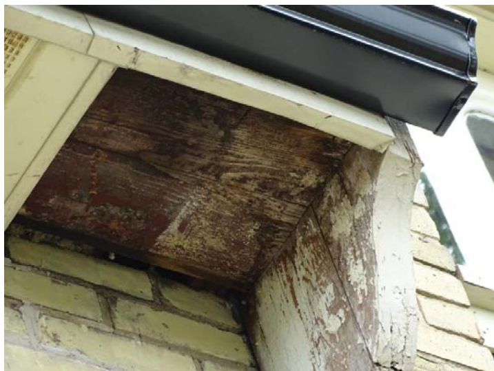
Figure 27: Missing Soffit Section along Front Elevation
