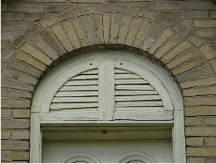
Figure 32: Exterior Transom/Shutter above Second Floor Door
