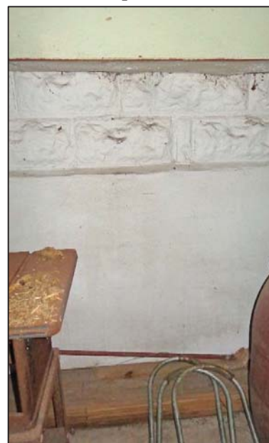
10. Room 16 – East wall, concrete block on poured concrete
