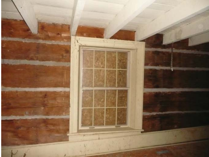
BEFORE: View of Interior showing modern replacement window, overhead floor joists, and exposed hand hewn logs with chinking
