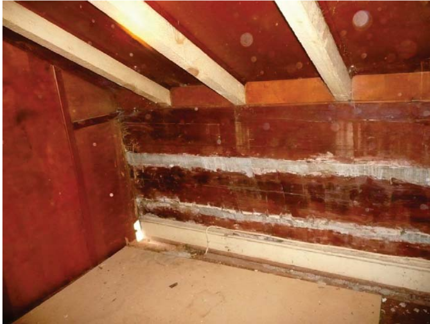
BEFORE: Interior view of hand hewn logs and ceiling joists (mezzanine).
