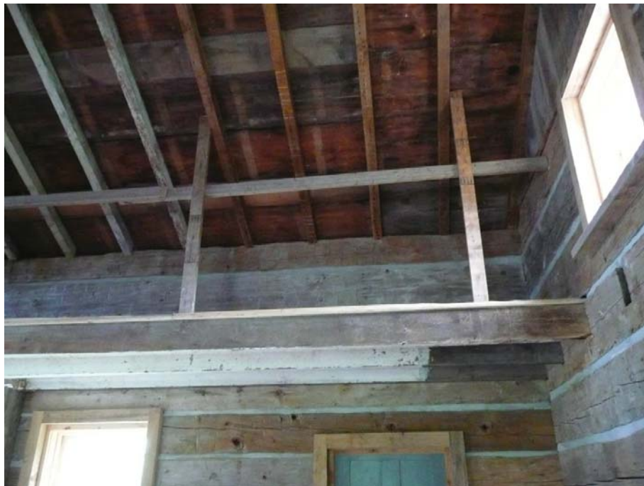
AFTER: View of Interior showing overhead floor joists, and exposed hand hewn logs with chinking.
