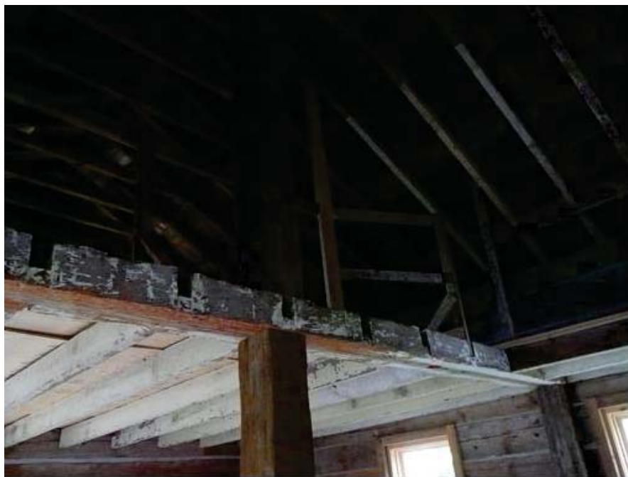
AFTER: Interior view of hand hewn logs and ceiling joists (mezzanine).
