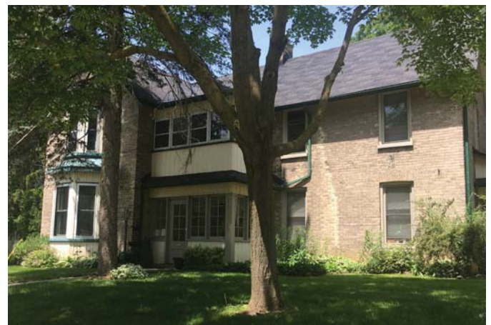
Dwelling's mass is broken through the articulation of the front elevation and the use of accent materials to emphasize the entrance portion
