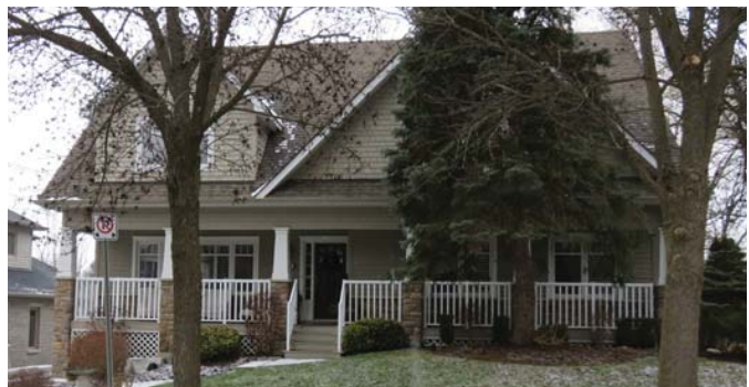
Wood clapboard as primary material with stone used as accent and metallic railings complementing the dwelling's architecture
