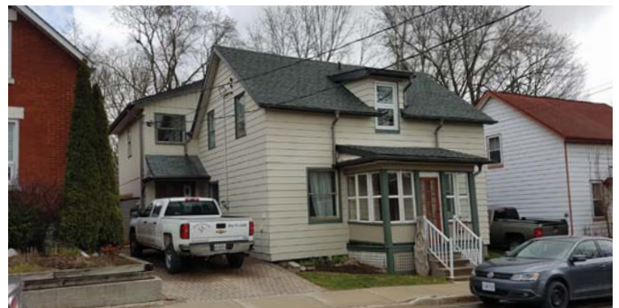
Extension to the back reflects scale and architectural proportions/details of original structure
