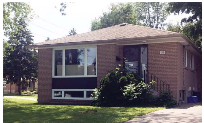
Example of a slightly recessed entrance feature covered by the main roof
