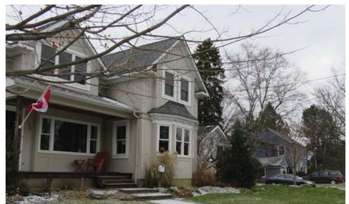
Articulated elevation with changes in plane and pitched roof lines
