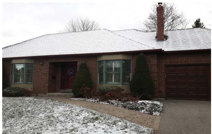
Low profile houses with shallow pitched roof lines dominate the Neighbourhood's built form
