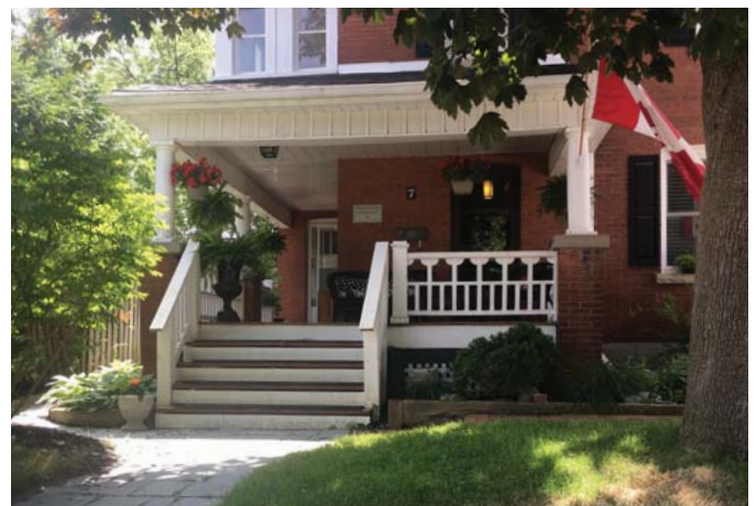
Articulated corner porch as main element of the front elevation
