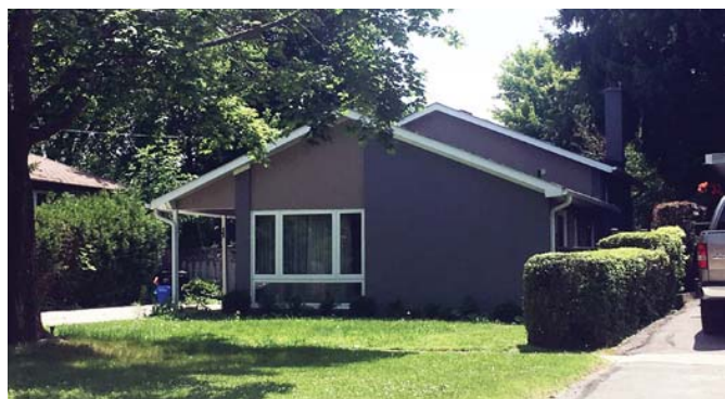
Shallow pitched roof lines complement simple building geometry
