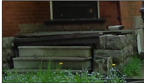
Figure No. 5.6 North porch base – foundation deterioration
