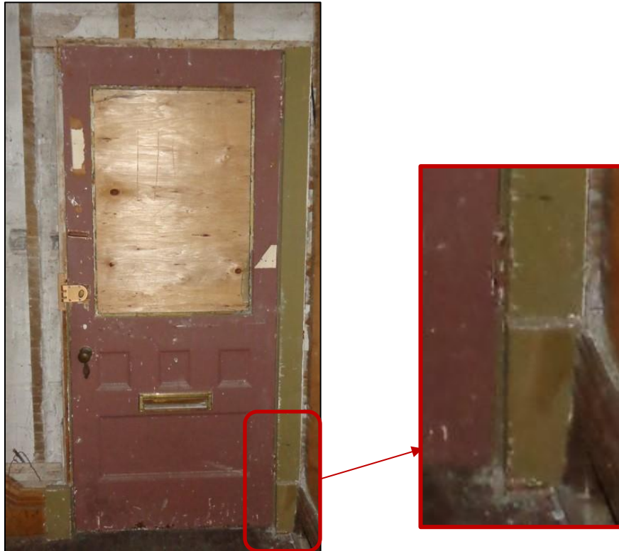
Figure No. 5.20 Front door, interior view showing remnant casing
